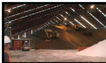
PDC Storage Shed 90000 tonnes
